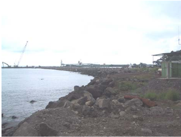
Figure 14. Sonara jetties and ship, next to the Oil Refinery at Limbe.
