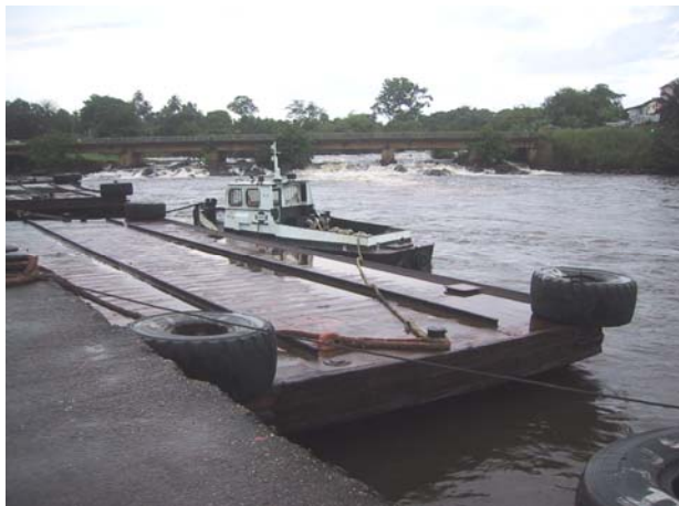
Figure 10. Kribi Port quayside, River Kienke and the road bridge.
