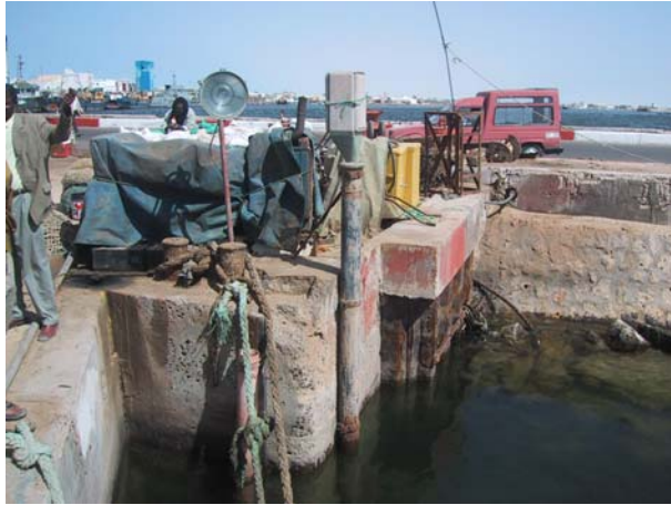
Figure 3. Nouadhibou Port Ott R16 Tide Gauge (no longer used).
