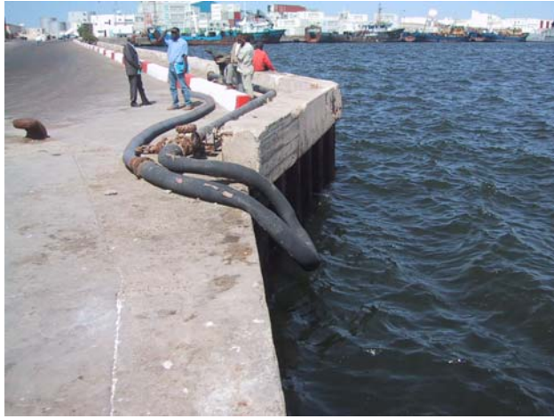
Figure 5. Location 1. Preferred site on North side of jetty for a tide gauge (to right of the IMROP staff).
