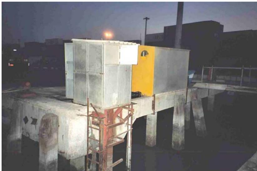
Figure 11. Float gauge (manufactured by the Ott company) in Bushehr.
