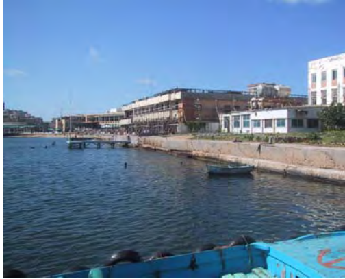
Fig.3. University of Alexandria, Oceanography Department (undergoing major renovations) adjacent to NIOF.
