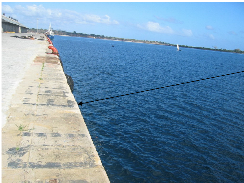
Fig 4: Mtwara Port main quay
