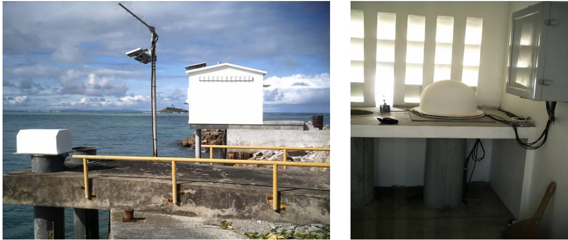
Fig 9: Building housing new tide gauge as part of the Indian Ocean Tsunami Warning System
