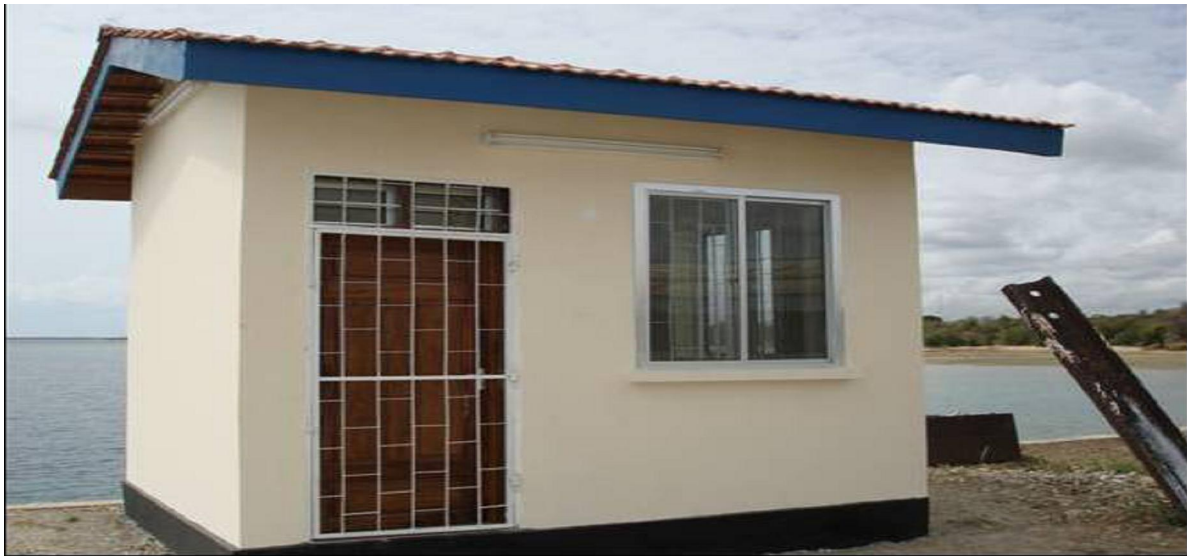
Fig. 3 Mtwara Port and the New Tide Gauge Hut
