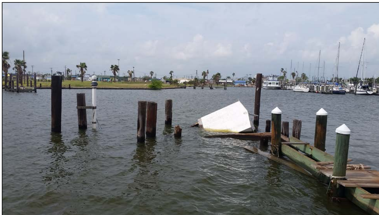
Figure 6. Rockport, Texas NWLON station after Hurricane Harvey
